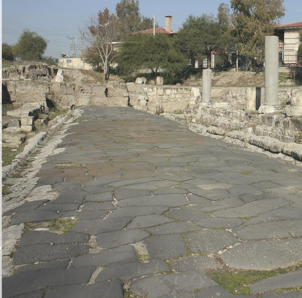
Tarsus: One of the main streets from the days of Paul. Note the basalt paving stones, white limestone curbing, and the remains of buildings that line the right side of the street.
